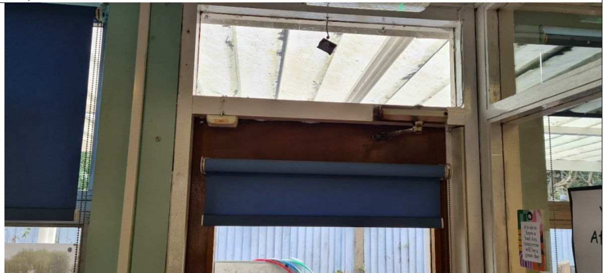
Example External Door to be replaced with mag sensors and door closer to be considered.
