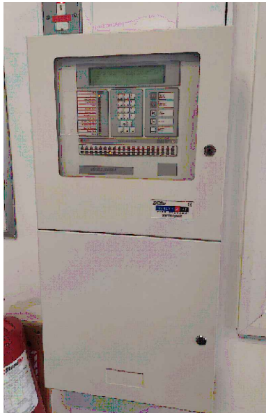
IMAGE 6: EXISTING FIRE ALARM PANEL
