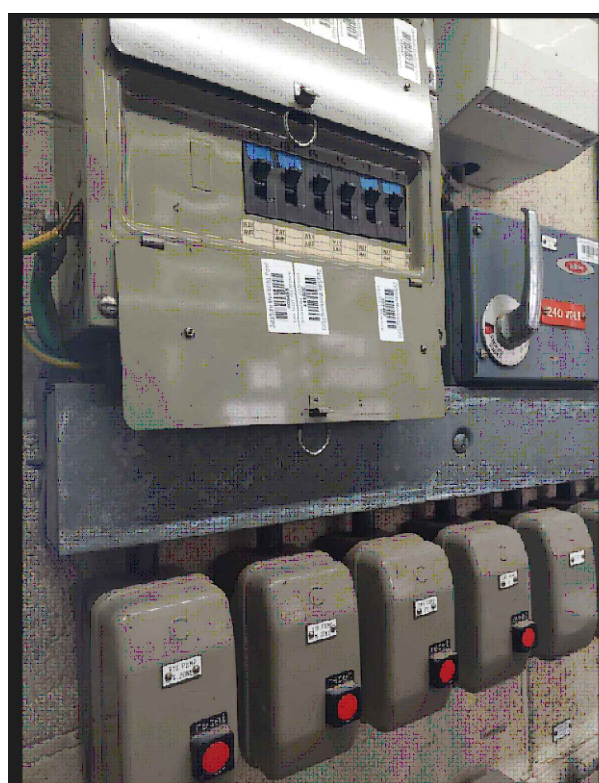
IMAGE 2: SP&N BOARD FEEDING EXISTING BOILERS
